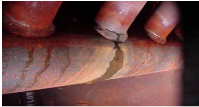
FIG. 2.4. Leaking tube to header welds provide multiple parallel leak paths.
